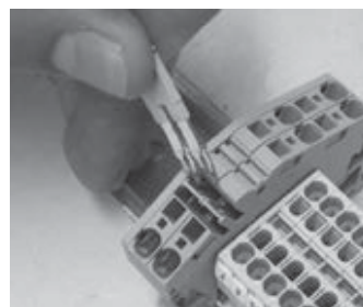
Removal of shunt to deactivate a heater (drop of 1000W)
